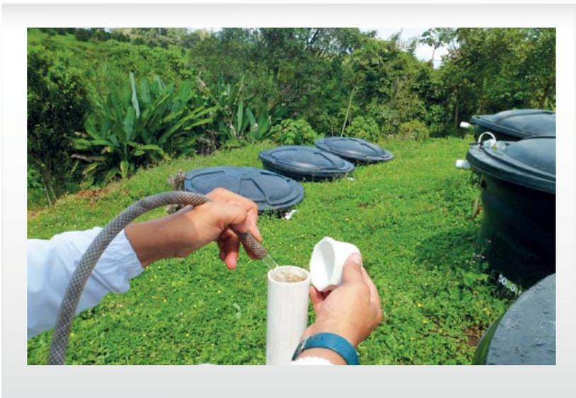
Figure 25. Purging of the system for sludge removal.
