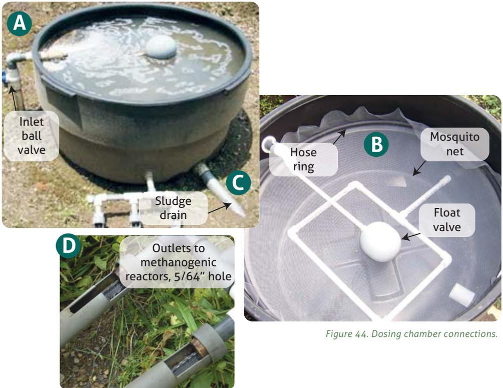
Figure 44. Dosing chamber connections.
