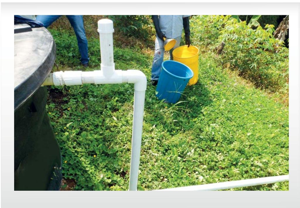
Figure 23. External pipeline or device for sludge removal.
