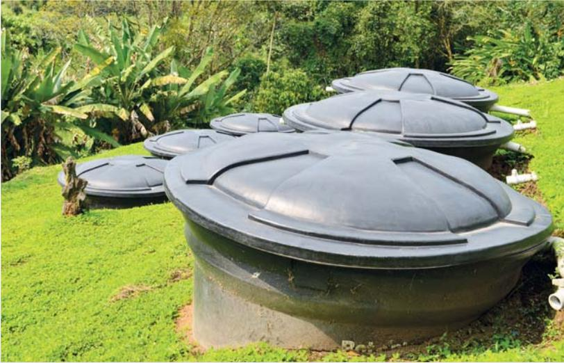
Figure 28. Half-buried anaerobic filters.
