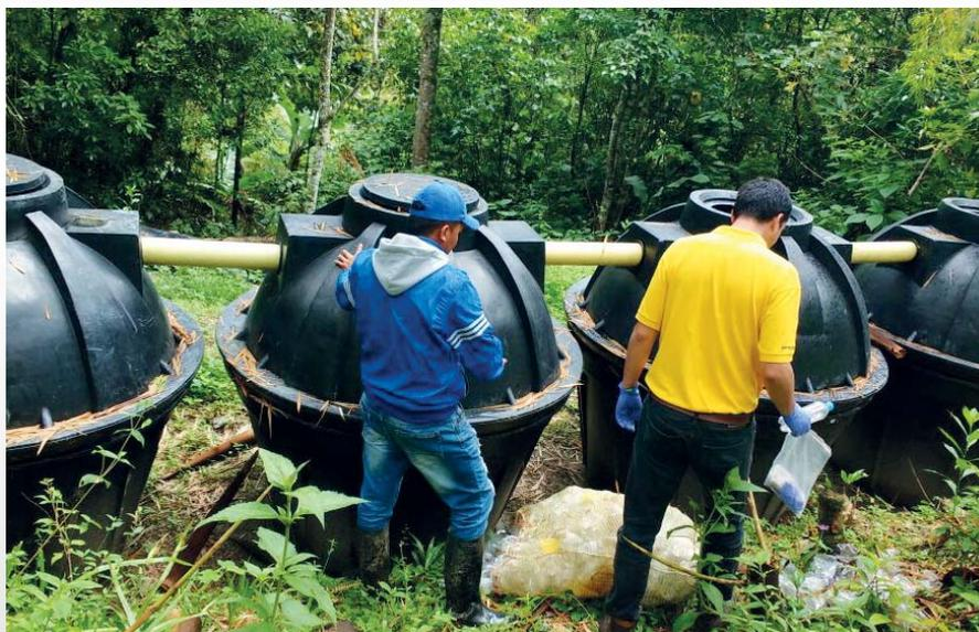
Figure 19. Septic tanks installed in the department of Cauca.
