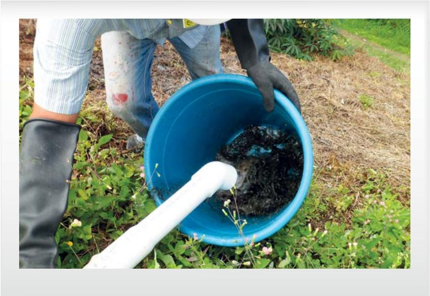
Figure 26. Sludge outflow.
