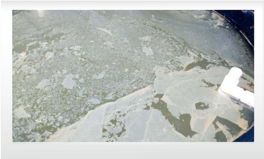
Figure 18. Appearance of floating grease in grease trap.
