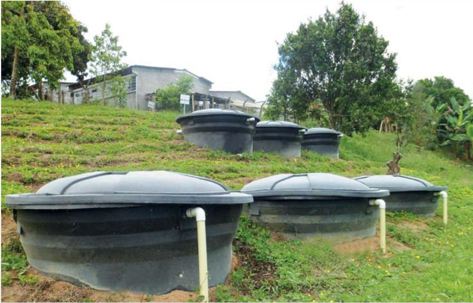
Figure 2.1. Half-buried septic tanks.
