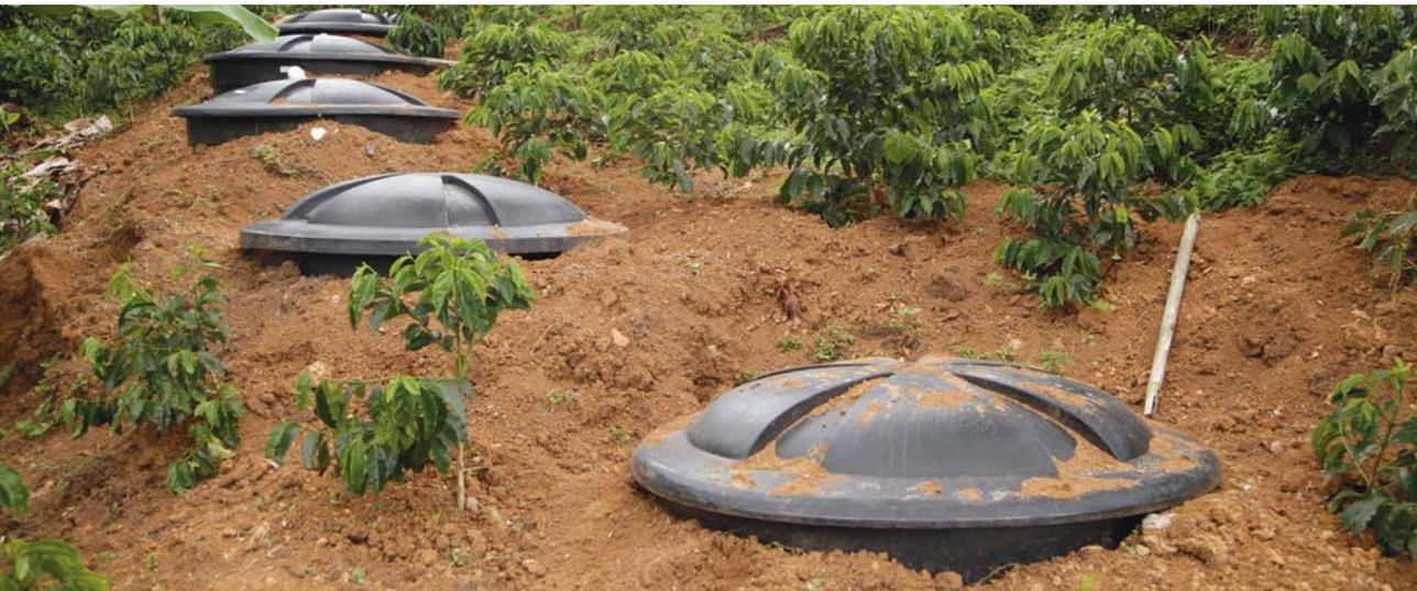
**Modular Anaerobic Treatment System**
